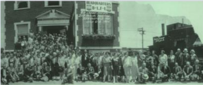
Commercial Club Building Restoration
