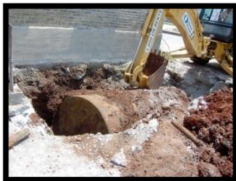
Removal of a UST, June 2005
